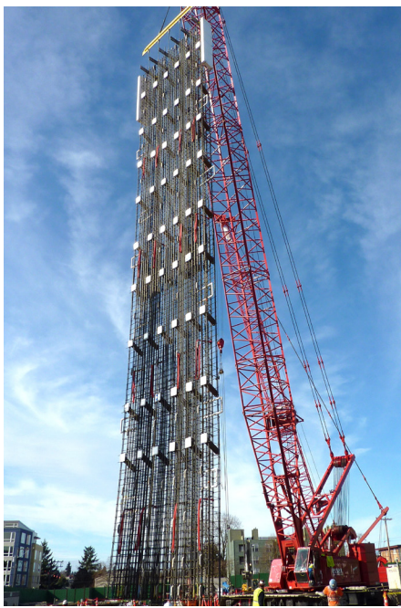
Rebar cage lift
